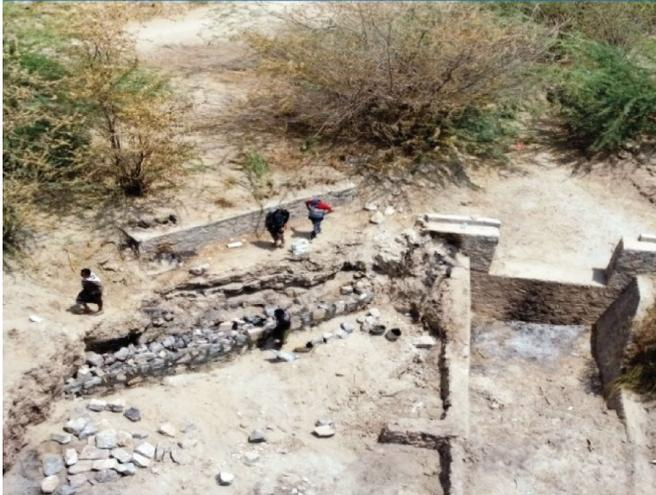
It includes restoring ditches No. 24 and 26, installing a 1.9-meter-wide and 2.5-meter-long iron gate, maintaining the protection wall, and cleaning the irrigation canal along 10 meters.
