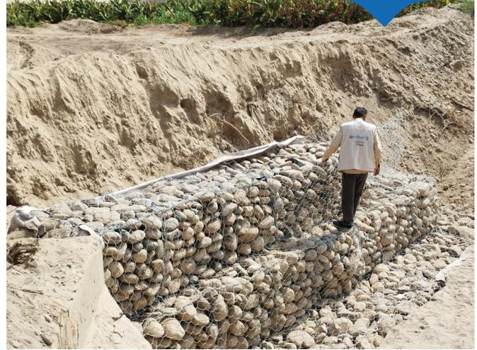
It includes constructing Al Mizan culvert, maintaining and restoring Al Mizan old ditch, and cleaning the irrigation canal from sesbania trees, sediments and dirt mounds.
