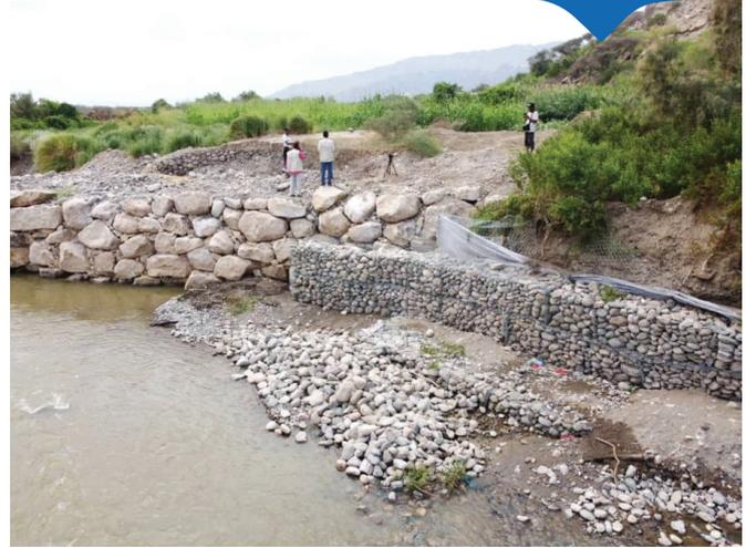
It includes removing sesbania trees, and cleaning sediments and dirt mounds from four canals in Amjablat Al Rahwi in Batis, with a length of 1540 meters, a width of 2 meters and a depth of 0.15 meters, requiring an agricultural tractor. It also includes constructing 48 of one-meter high and 24 of fifty-centimeters high sand gabions next to the new culvert.
