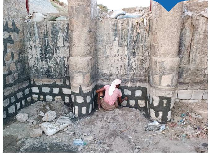
It includes comprehensive maintenance of the iron gates of ditch No. 2 Arshan, and the gates of ditches No. 3 and 5, and removal of sediment deposits in front of the gates and the ditch and on both sides of the canal with a length of 500 meters, a width of 4 meters and a depth of 0.5 meters. It also includes restoration of the ditch using cement and stones, and removal of waste and trees on both sides of the canal with a length of 450 meters and a width of 3 meters and a depth of at least 15 cm.
