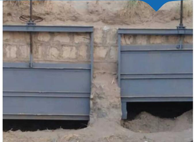
It includes restoring the main gate, 2.7 meters wide and 2.5 meters high, and maintaining the culvert and covering it with a 10 cm thick plain concrete protection layer.
