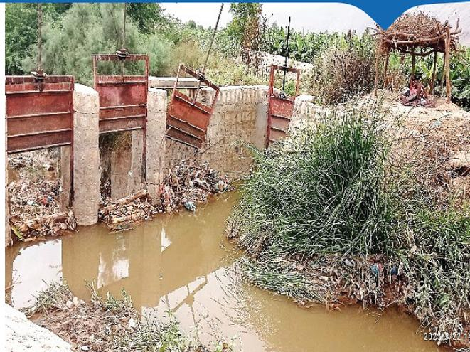
It includes cleaning the canal from sesbania trees and sediments, restoring the stone structure of the culvert, and maintaining the iron gates.
